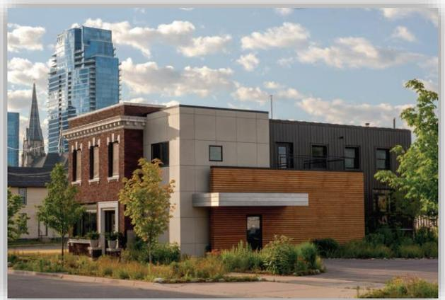
The renovation of the nearly 4,000 square foot LEED Platinum building, completed in March 2010, enables the repurposed building to use 60 percent less energy than a typical office building, 45% less water than the expected baseline, uses a typical market rate of \$125 per gross square foot, has zero storm water discharge, and provides a native landscape habitat for a wide variety of birds and insects.
