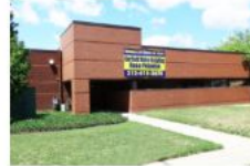
Garfield Metro Building
